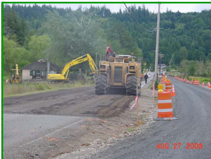
During East Quilcene Rd reconstruction, a temporary bypass (shown on the right in the photo above) was opened to accommodate thru traffic while work continued on the road.
