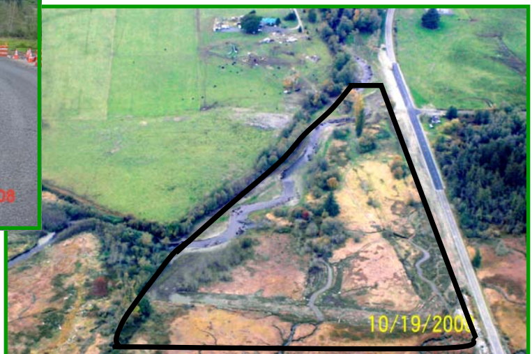
Public Works acquired this flood-prone property in 2000 using grants and worked cooperatively with HCSEG on the restoration project.
