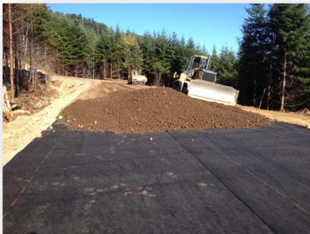
Spreading gravel base over geotextile for subgrade stabilization of the new road.
