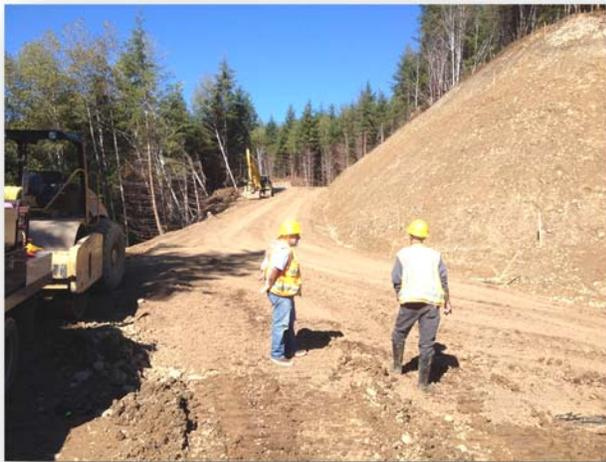
This 35-foot high, cut slope required moving 20,000 cubic yards of earth.
