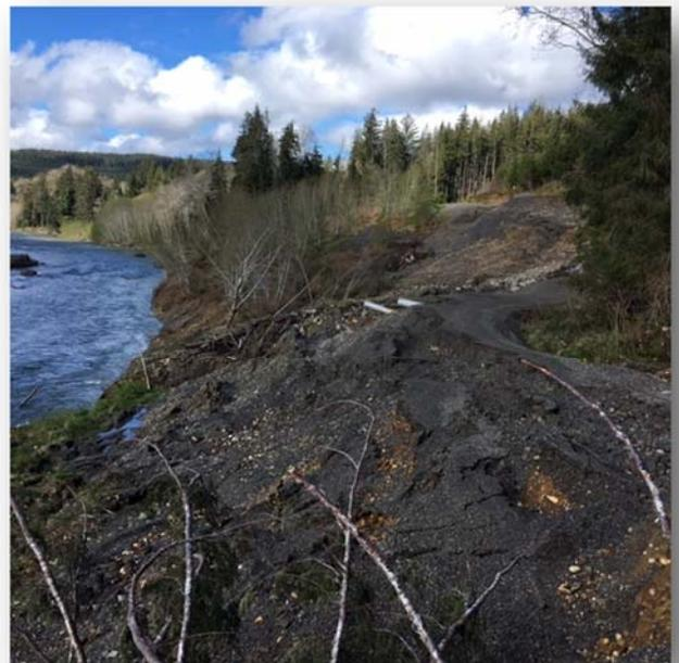
The original Undie Road is barely recognizable as it continues to slide into the Bogachiel River. Notice the two culvert pipes protruding from what remains of the road surface.
