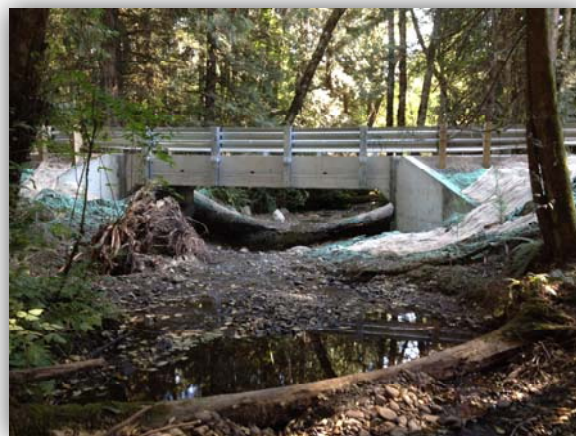
Once the new culvert was installed, the streambed was reconstructed.
