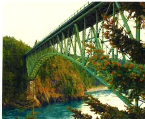
SR20 Deception Pass Bridge
