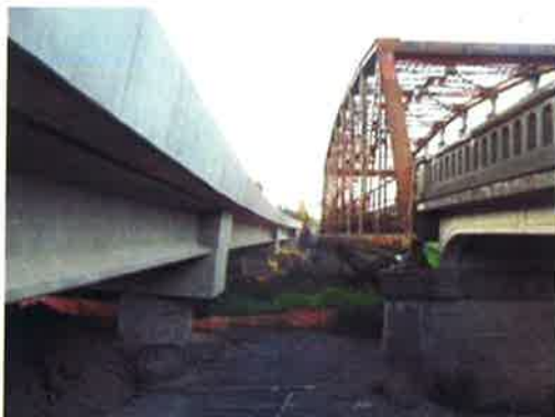
SR6 Wiliapa River bridge
