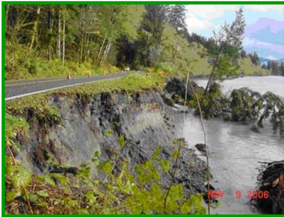
Flooding of the Hoh River washed away the river bank adjacent to the Upper Hoh Rd – in some places to within less than a foot away from the road. The river bank that remained after flooding was unstable.
