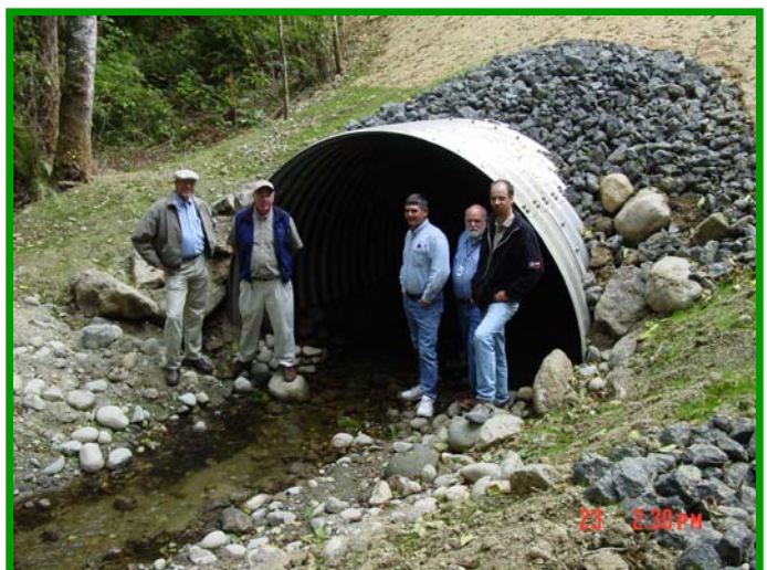
HCSEG and County staff stand by new culvert at Dabob Rd.
