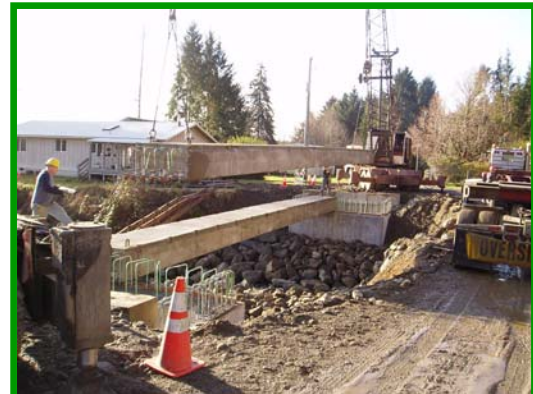
New pre-cast bridge slabs being placed.
