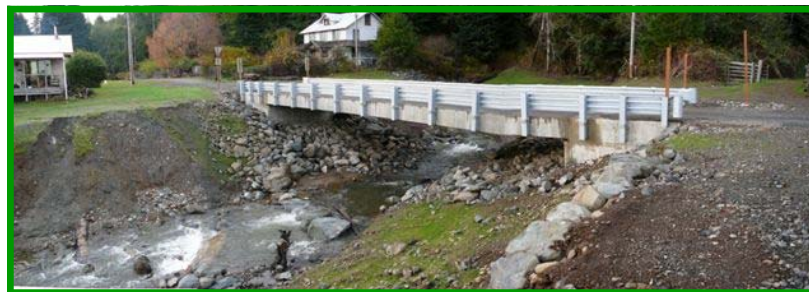
The new bridge provides a much wider opening for Fossil Creek.
