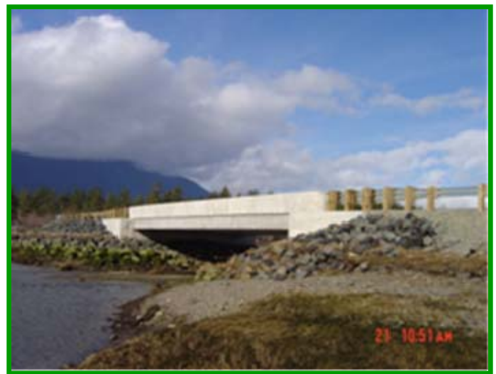
The new bridge over Donovan Creek removed an intermittent fish barrier and allows more natural estuary conditions to develop on the north side of East Quilcene Rd.
