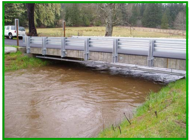
The new bridge easily handles a high flow event.
