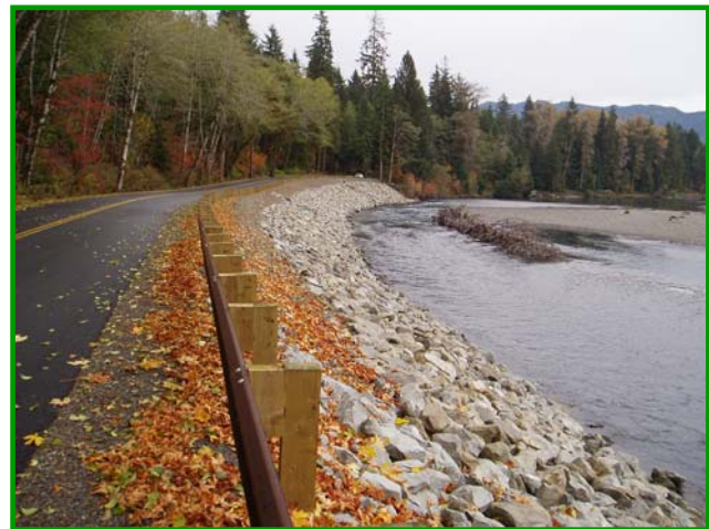
Upper Hoh Rd at milepost 7.8 after repair completed in October, 2008.
