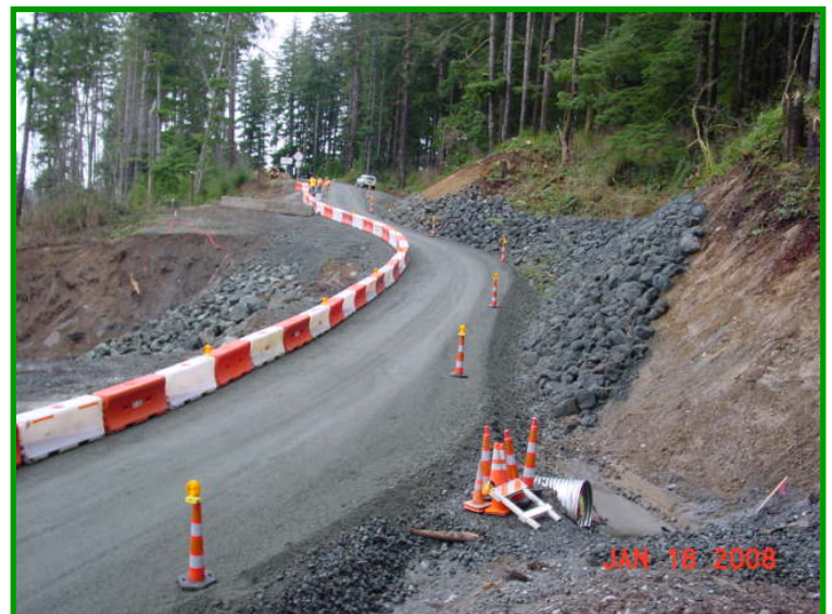
Dowans Creek Rd after repairs on January 18, 2008.
