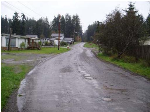
Before improvements on 6th Ave, the uneven gravel surface, dust, potholes, and poor drainage were problematic.
