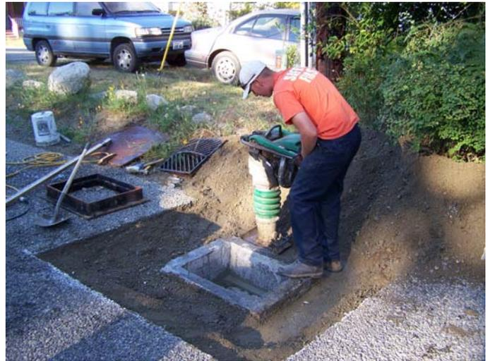
▲ Improving drainage was an important component of this project. In this photo, Corey Woodley compacts backfill material around a new catch basin.
