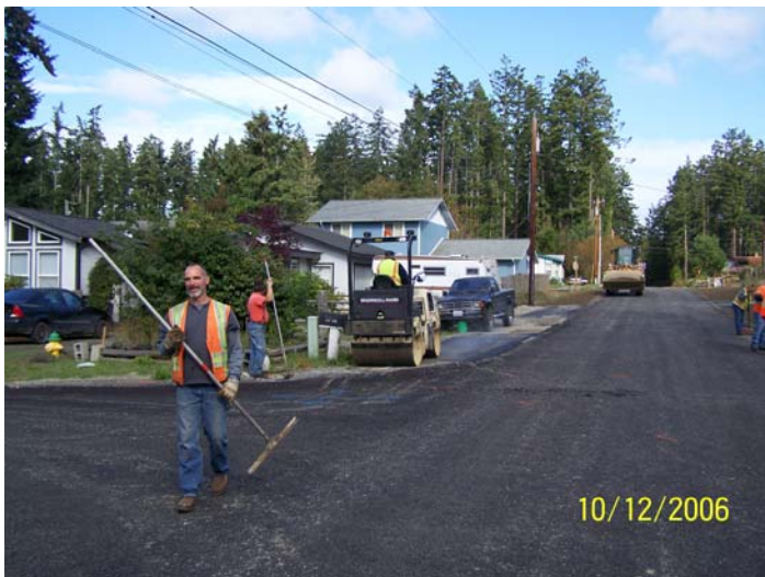
▲ Asphalt is applied by hand to driveway approaches to ensure a smooth transition from the street. Tom Borges and Dale Brownfield spread asphalt on this approach while Richard Liske operates a roller, compacting the asphalt.
