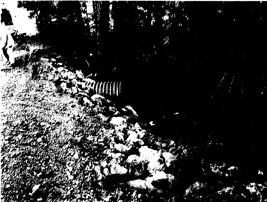
After repairs – November 27, 2012
