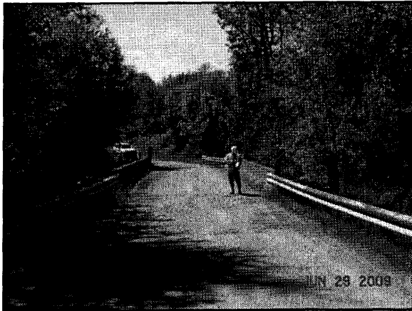
Bridges are inspected at least every two years pursuant to State rules.
